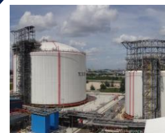
Low-temperature tank terminal completed in Singapore in 2015
