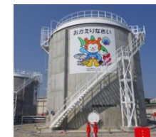
Completed construction of Japan's first five tsunami-resilient structured tanks in Kesenumma, Miyagi in 2020
