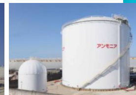
Completed construction of Japan's largest low-temperature ammonia tank in 2022
