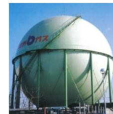
Completed construction of one of the Japan's largest city gas holders in 1995
