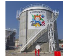
Completed construction of Japan's first five tsunami-resilient structured tanks in Kesenumma, Miyagi in 2020
