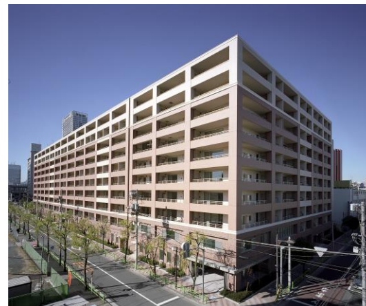
Exterior view of Residence Charmant Tsukishima
