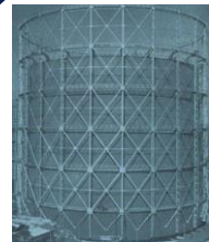
Largest wet seal gas holder in East Asia (at that time)
