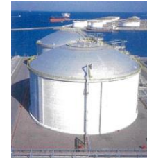
Low-temperature tank made of PS concrete. Received many authorized certifications, including the Technological Progress Certification from the JPI (Japan Petroleum Institute) in 1978
