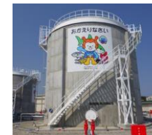
Completed construction of Japan's first five tsunami-resilient structured tanks in Kesennuma, Miyagi in 2020
