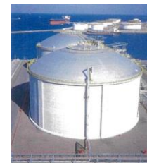
Low-temperature tank made of PS concrete. Received many authorized certifications, including the Technological Progress Certification from the JPI (Japan Petroleum Institute) in 1978
